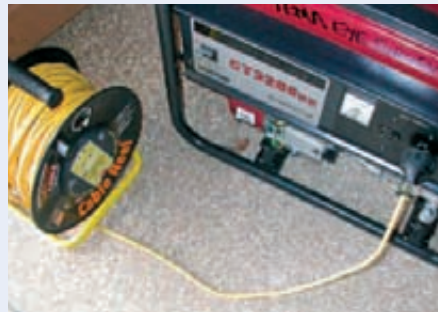
Figure 1. Connecting the cable reel to the generator. Note: unroll the cable reel before you plug the voltage regulator into the cable reel socket
